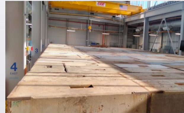
June 2022: overburden complete
