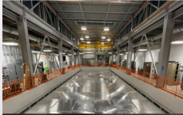
Dec. 2021: CRT installation complete
