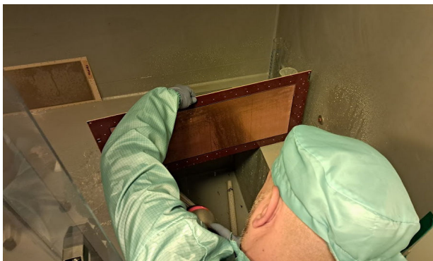
Low pressure cleaning with DI water
