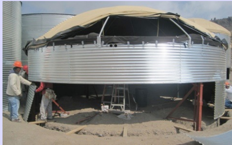
Steel frame construction
